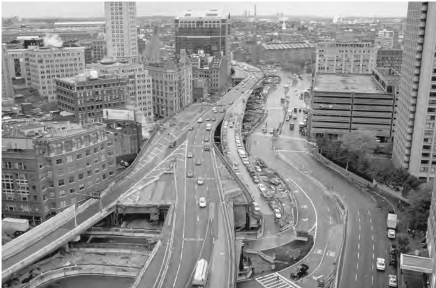
1-2 The site of the future Wharf District Park. The elevated multilane highway, affectionately known as “the green monster,” had separated the city from its waterfront since the 1950s. © 2005 by EDAW. Photograph by Dixi Carrillo.
